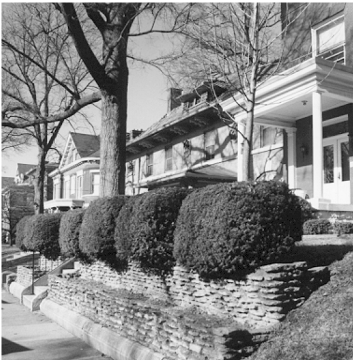
Gently-sloped front- and side-yard berms and concrete and limestone curbing are historic features on many blocks and should be not back-filled or terraced.
