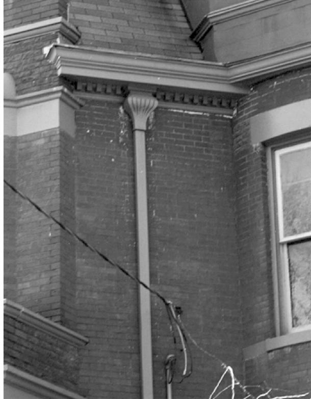
*Gutters, in combination with flashing and downspouts, help quickly move water off the roof and away from the building. Clogged, deteriorated, or missing pieces will cause the gutter system to fail, which will lead to moisture-related deterioration.*
