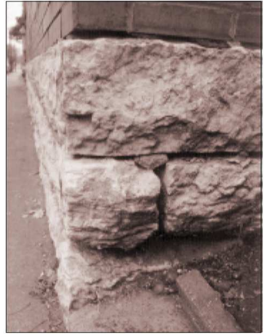
Moisture often enter walls from the base. Repeated freezing and thawing have crumbled the mortar at the foundation level of this structure.
