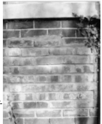
*Where bricks are not "toothed-in" to the original masonry, patches are obvious.*
