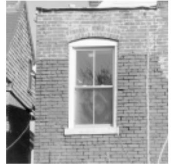
Mortar bonds masonry together, permits movement, and acts as a conduit for moisture transpiration. Walls, such as the one seen above, that have damaged or inappropriate mortar are at risk of freeze-thaw deterioration.
