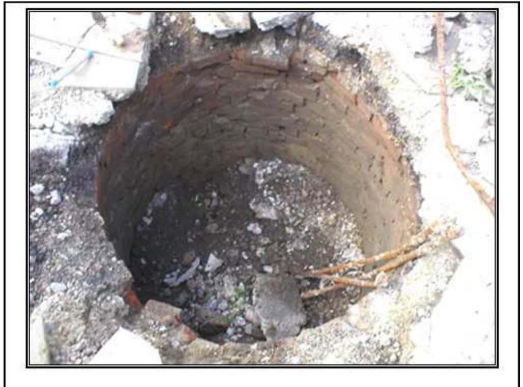
A privy found under a concrete parking pad on Pope Street. A property owner discovered and reported this privy. After proper assessment, it was filled in and the construction project was completed.
