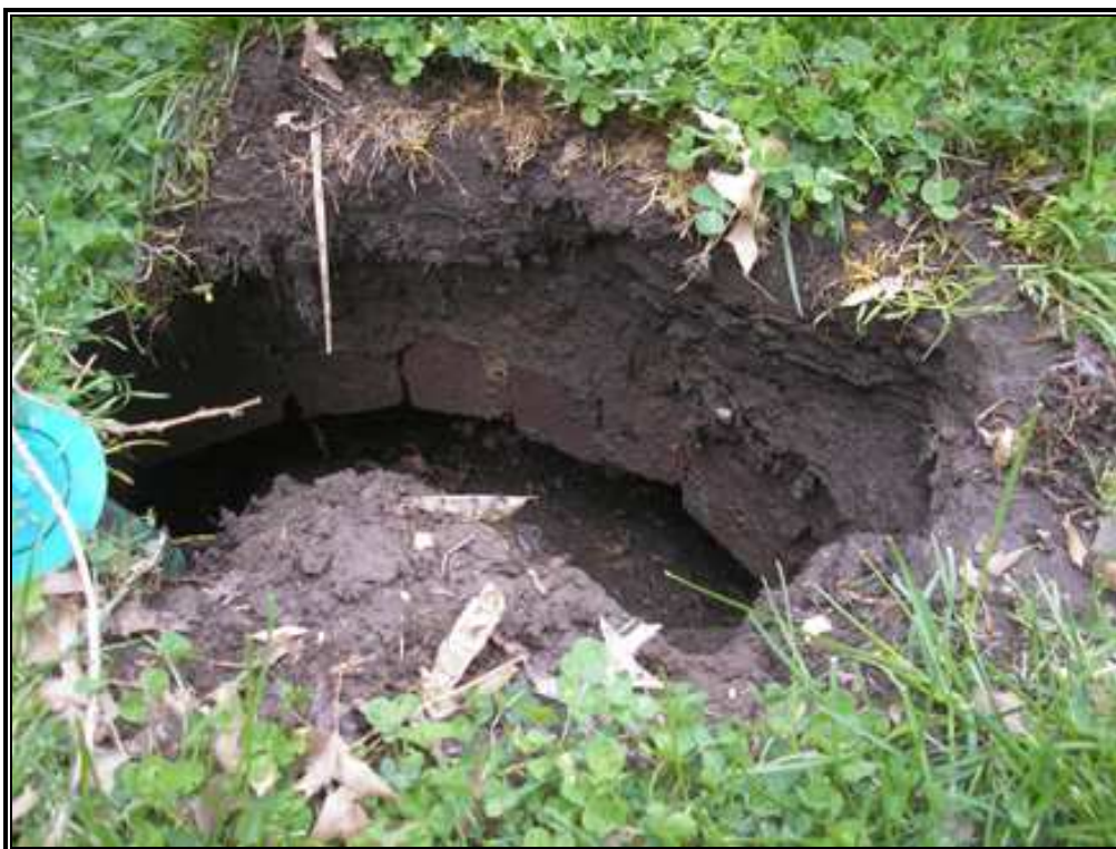
A water cistern found in a yard on Pope Street.
