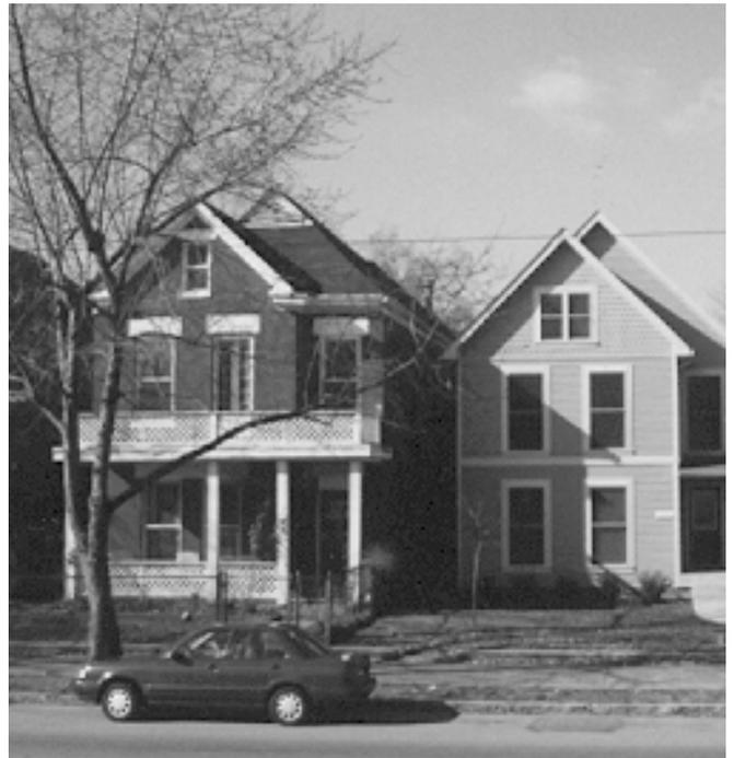
*New construction (right) is a close match to historic construction (left). Frame construction is appropriate for this block, which contains a mix of masonry and wood houses.*
