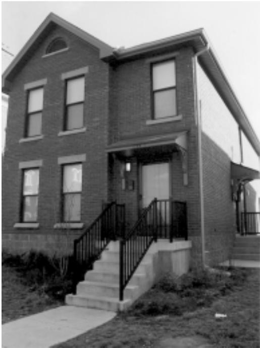
*This new building incorporates a number of historic features into a modern, yet traditional, design: slightly-projecting facade, raised foundation, contrasting lintels and sills, masonry construction, and covered entry.*
