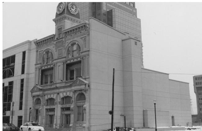
*The elevator tower on the German Insurance Building is an example of a successful addition. It blends in with the side facade and does not attract undue attention.*
