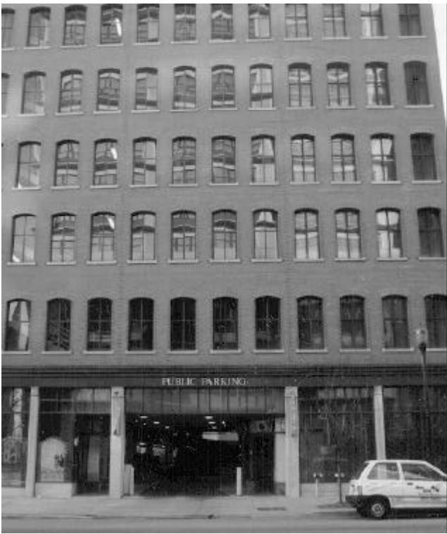
This West Main Street parking garage uses historically-inspired facade elements to blend in with its neighbors.
