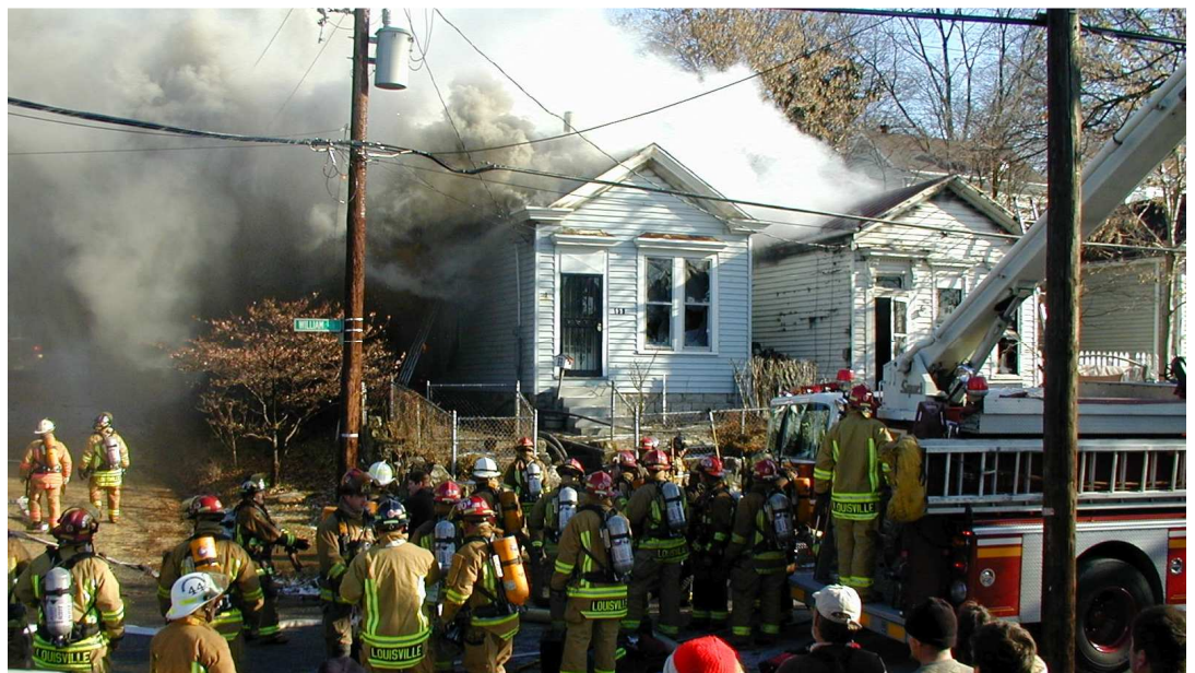
Only due to a safety threat posed by serious structural damage, such as that caused by a major house fire like this one on William St., will officials issue an Emergency Demolition Order.
